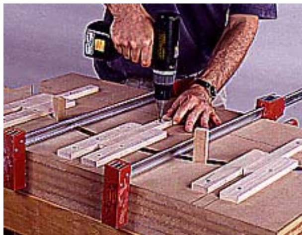
3 Use 3/4-in.-thick spacers between the bending form pieces. Clamp the form pieces together and fasten alignment strips.
