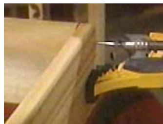
Use at least two screws to attach each corner together
