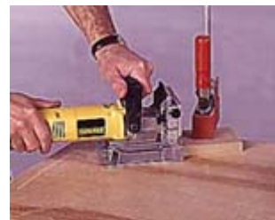
5--Cut plate slots in the grid assembly components. Clamp pieces to your work surface for safe and accurate cuts.
