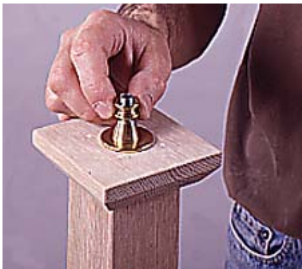
10--Slide the brass check ring over the steel pipe. Then thread on the tapered coupling, steel nipple and brass spindle.
