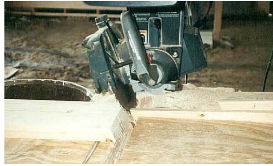
Sawing the fly rafters
