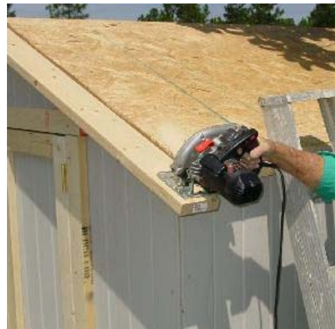
Trimming the Fly Rafter
