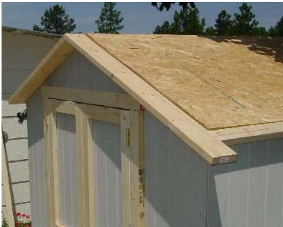
Installing the Fly Rafters
