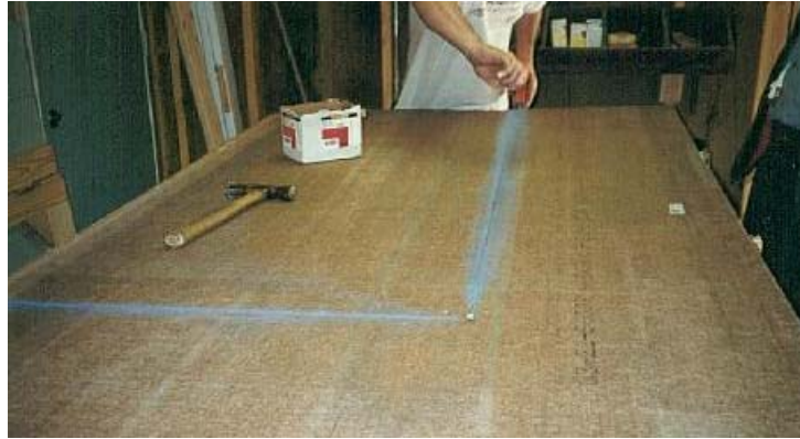
Cut through the back of the siding at the top and side of the door.
