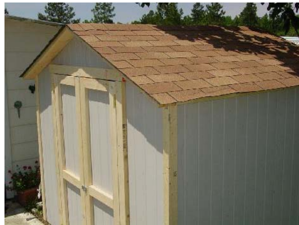
Finished and ready to paint.
