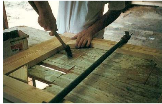
Nail the corner blocks in place.
