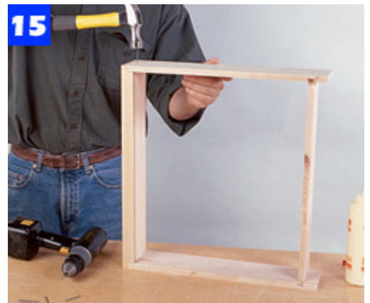
Bore pilot holes through the drawer sides, then use glue and nails to assemble the drawer box.
