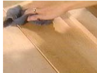
Wipe off excess with a rag
