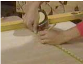
Mark out two 38 inch by 24 inch rectangles
