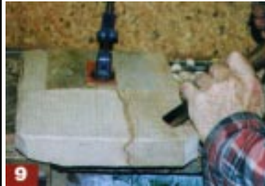
Using the chisel across the grain
