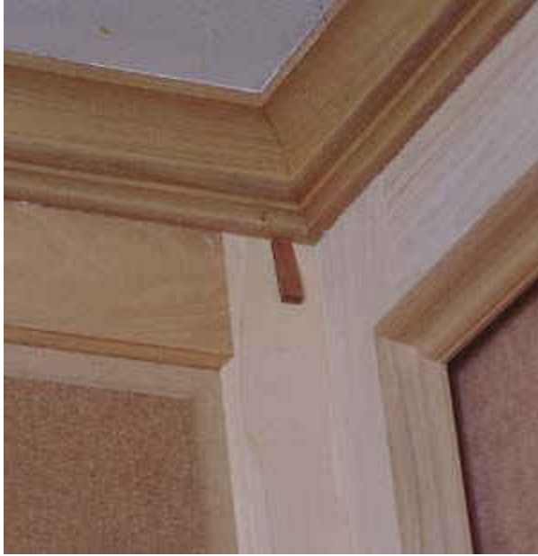
Photo 12- Use small pieces of door shim (available at lumber yards and home centers) as wedges to push inside miters together. Tap in with a hammer. When the glue dries, cut the shim off, don't pull it out.
