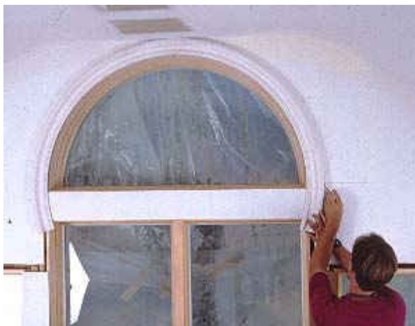
Photo 15- Mark out half round moldings by scribing a straight line on the wall, aligning the molding to the line, and marking the curved mold on both sides where it intersects.
