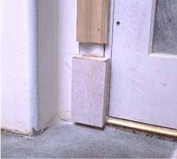
Photo 2- Glue vertical molding to plinth
