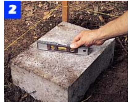
Dig a hole for the first block at the highest point in the grade. Add gravel, install the block, align it with the string, and level it.
