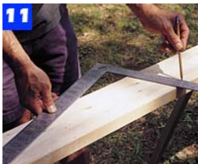
To find the rafter cutting angle, align the 5- and 12-in. marks on the framing square's legs with the edge of the rafter stock.
