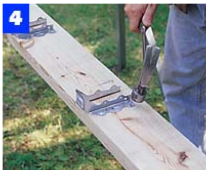
After marking joist locations on long front and rear rim joists, install metal hangers with 1-1/2-in. joist hanger nails.
