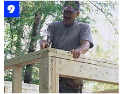
Frame and raise the remaining walls without sheathing. After nailing together the corner studs, add the top plates.
