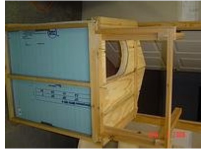
Figure 2. Underside of house and deck frame.
