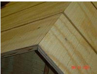
Figure 5. Close-up view of roof joint.
