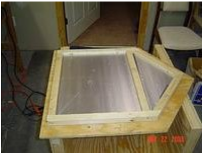
Figure 6. Back wall with framing and insulation in place.
