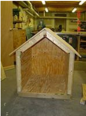
Figure 4. Side view of roof with front wall removed.
