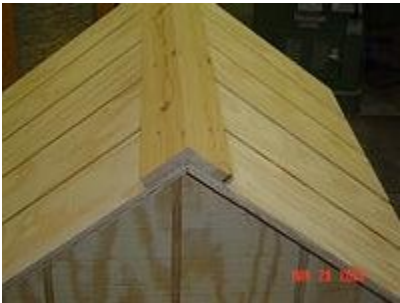
Figure 11. Ridge cap in place.
