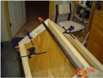
Figure 3. Test fitting rafters.
