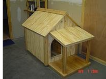
Figure 5. The finished deck and deck roof.
