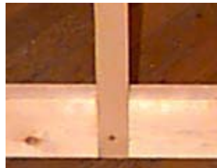
fig. 3: bottom brace with chiseled center support recess
