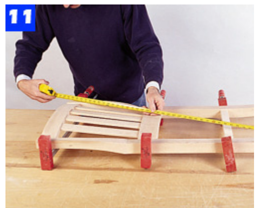
Join the back rails to the rear legs and clamp. Compare opposite diagonals to check that the assembly is square.
