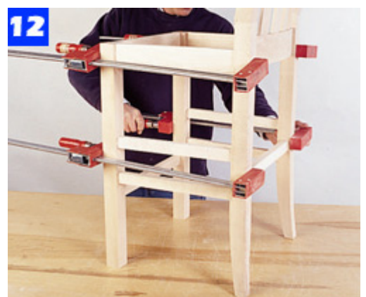
Join the rear and front subassemblies with the side rails. Set the stool on a flat table to check that the legs are even.
