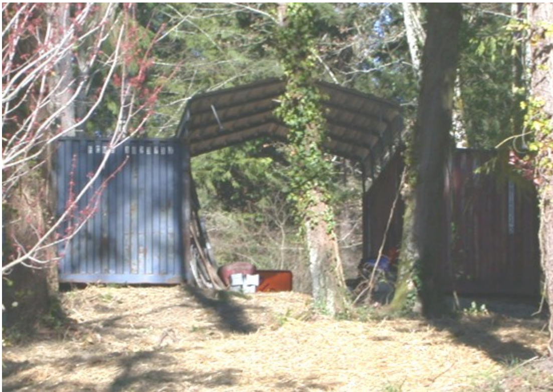
Carport made with two, twenty foot containers and bridged aluminum covering.
