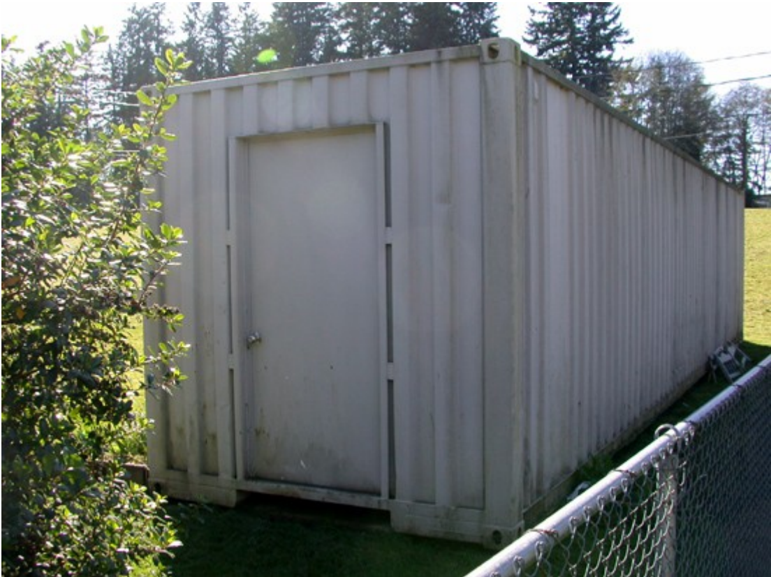
Forty foot container utility building with basic door addition.
