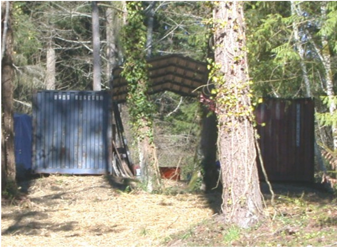
Carport made with two, twenty foot containers and bridged aluminum covering.
