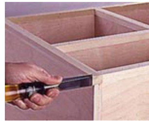
8--Use a chisel to cut a small clearance notch in the top corner of each vertical facing strip. Cut in toward the case.
