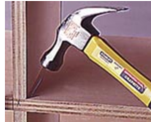
7--Drive finish nails at an angle through the tall partitions and the middle shelf, and into the short partitions.
