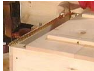
The overhang on the lid should be even on the front and sides.
