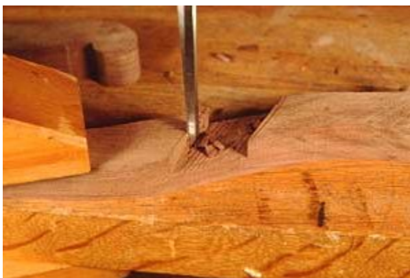
Photo 13- Fine tuning the lap walls with a chisel.
