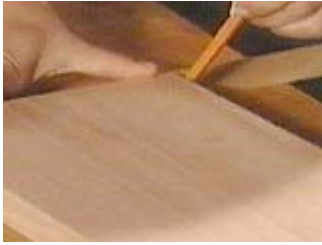
Hold the panel molding in place and mark for cutting
