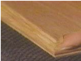
Use oil-based wood filler to fill any voids
