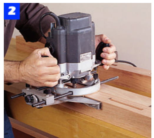
Lay out the mortise positions in the posts, and use a router with a straight bit and edge guide to cut the joints.
