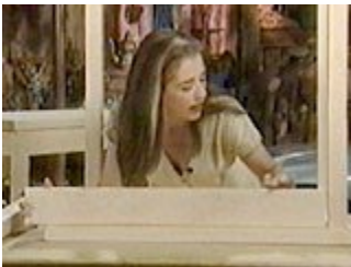
Put the apron lumber in place and mark it for cutting
