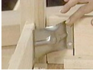
Cut the slots for the leg braces
