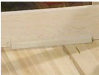
Make one-inch strips to support the apron
