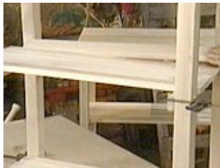
Space the shelf boards evenly and screw them down
