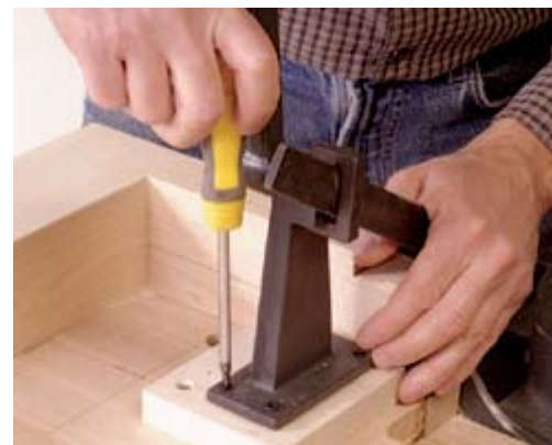
13 Secure a mounting block under the benchtop to support the tilt bracket for the side vise.
