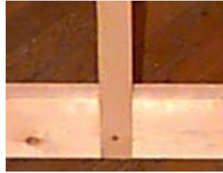
fig. 3: bottom brace with chiseled center support recess
