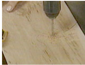
Drill holes as necessary to help start the blade
