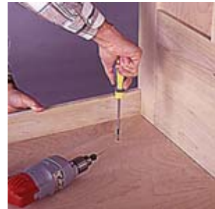
19--Place the platform assembly on the storage unit and tight against the headboard. Secure the platform with screws.
