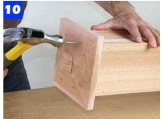
Position the cap so it overhangs the post uniformly. Then, fasten it to the top of the post with galvanized finish nails.
