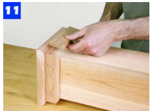
Miter the ends of the cap molding pieces. Fit each piece under a cap and secure with galvanized finishing nails.
