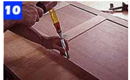
Use a chisel to outline each mortise. Then, make a series of cuts across the grain and about 1/8 in. apart within the waste area.
