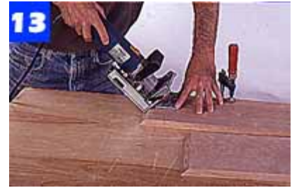
Cut the base pieces to finished length with mitered ends. Use joining plates in the miters to help hold the joints tight.
