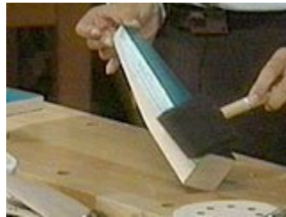
Remove any excess quickly with a dry sponge brush
