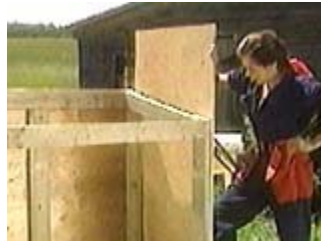
To mark the angle hold the plywood in place and mark
