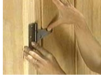
Attach hinges to the doors and the side trim
