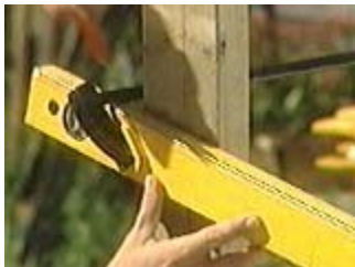
Clamp a straight edge on the front post and experiment with the roof pitch
