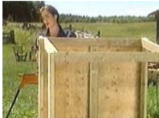
Use the plywood to square up the framing as you go
