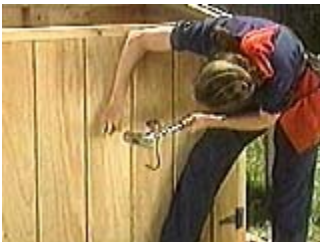
Attach closing hardware to the doors
