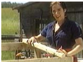
The angle for the rafters is the same as the one cut on the side posts
