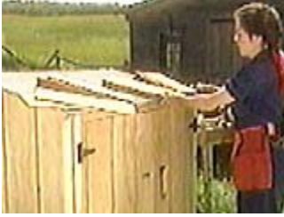
Separate the cedar shingles into their various sizes
