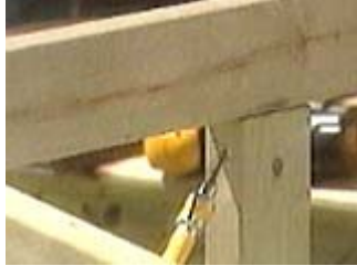
Toe-screw a center support to the back
