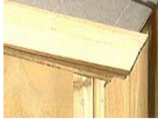
The two layers should overlap the front and sides by about half an inch
