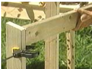
Use clamps to balance the boards while attaching them
