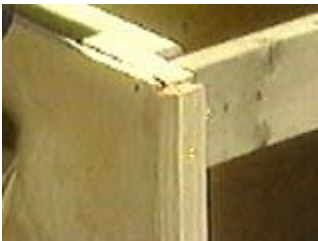
Attach 1x2 trim on the front sides and along the top
