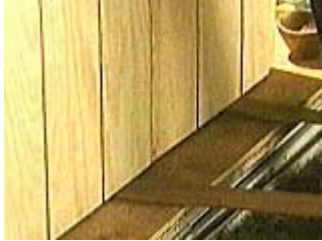
Use shims to hold the doors square in the opening
