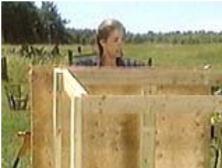
Cut and attach the plywood to the back and sides
