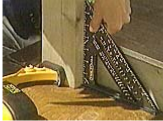
Square them to the floor
