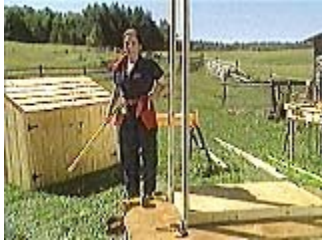
Clamp two long 2x4s to one end of the floor
