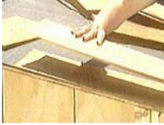
The first row of shingles should have two layers
