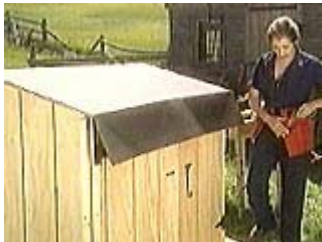
Attach the top with hinges and cover with 15 pound tar paper roofing felt
