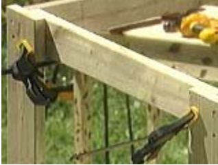
Attach using three inch zinc screws
