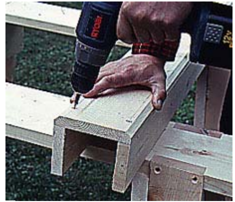
5--Assemble three-sided post boxes. Bore screw pilot holes and drive screws at a slight angle so heads miss the post chamfers.
