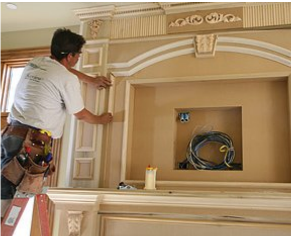
Cutting the flex molding and finishing up the trim on the face of the overmantel.
