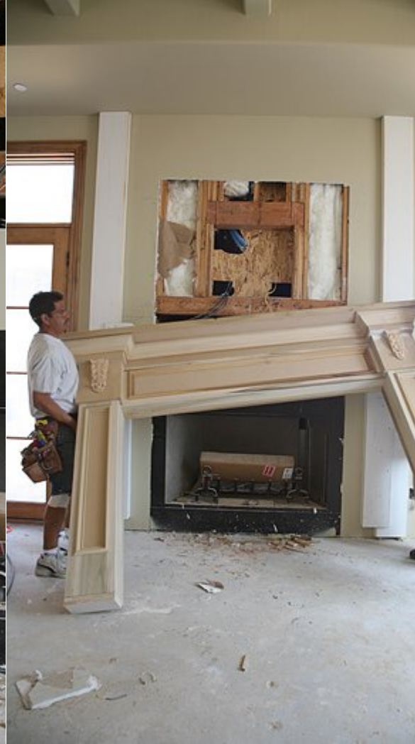
Then moved the lower mantel into position.
