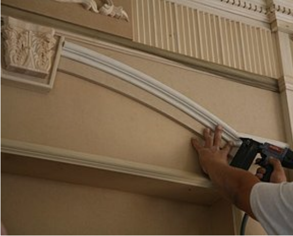
Cutting the flex molding and finishing up the trim on the face of the overmantel.
