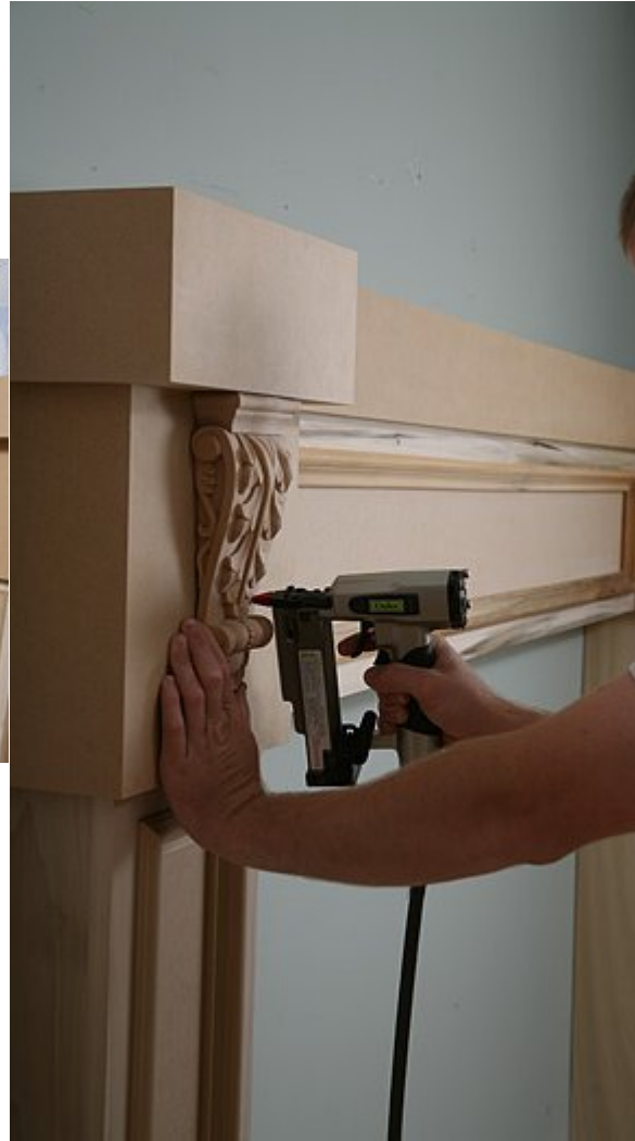
The bed band for the lower mantel went on next, then the lower corbels.
