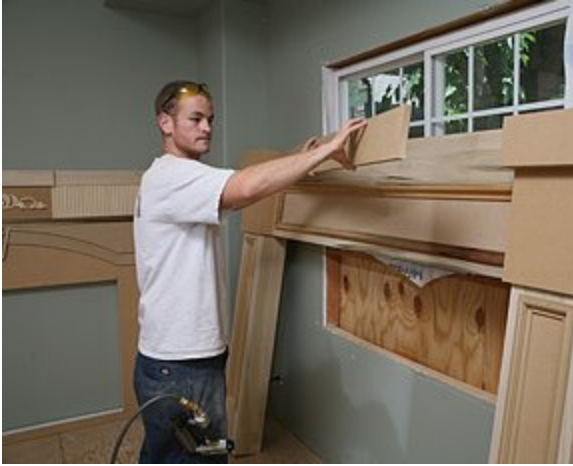
The bed band for the lower mantel went on next, then the lower corbels.
