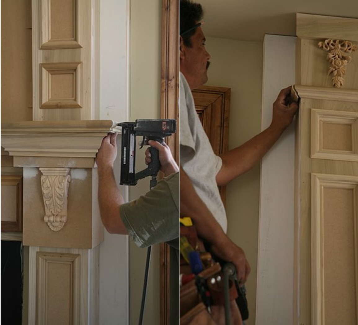
All that remained was applying the trim, starting with the self returns.
