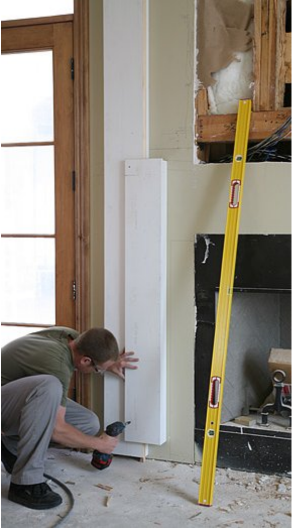
Next we installed backing for the lower mantel pilasters.
