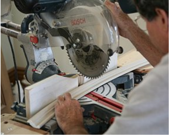
Cutting the flex molding and finishing up the trim on the face of the overmantel.
