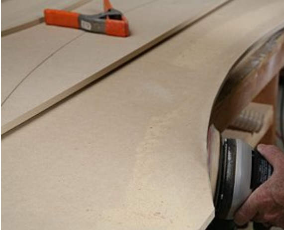
The arches didn't have to be perfect, just close for the panel molding, so I sanded to the trammel mark.
