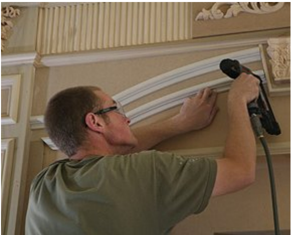
Cutting the flex molding and finishing up the trim on the face of the overmantel.
