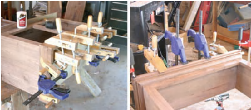
Left: Install the bottom aprons with glue and screws from the back side.
