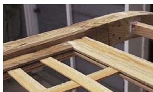
The panels are constructed out of channels made of wood that are attached to the side rails and corner posts. The lattice strips are inserted into the channels.
