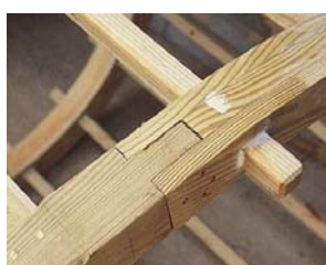
For strength and stability, the arch of the arbor is attached to each corner post with an open mortise and tenon joint.
