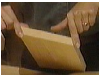
To fit properly, the board profile should be a parallelogram
