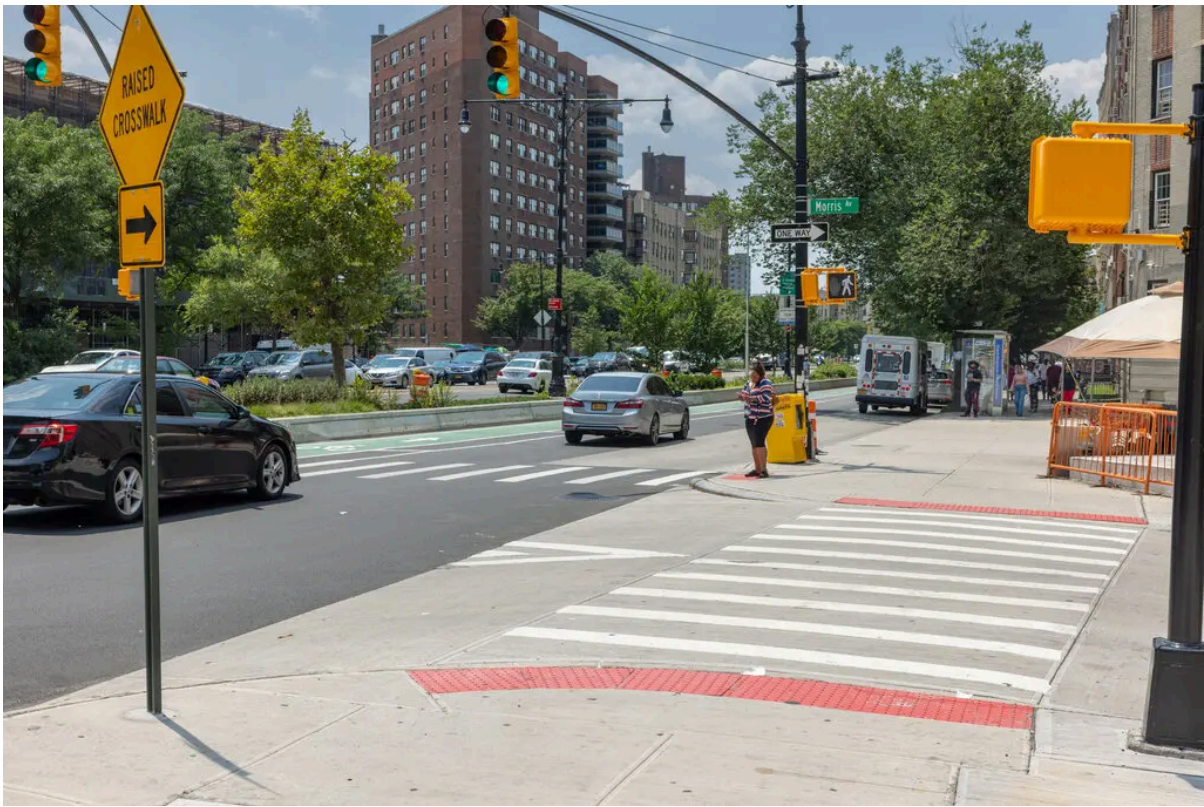
Raised crosswalks, like this one in the Bronx, have been proven to make streets safer for pedestrians. Matthew Lapiska/Department of Design and Construction
