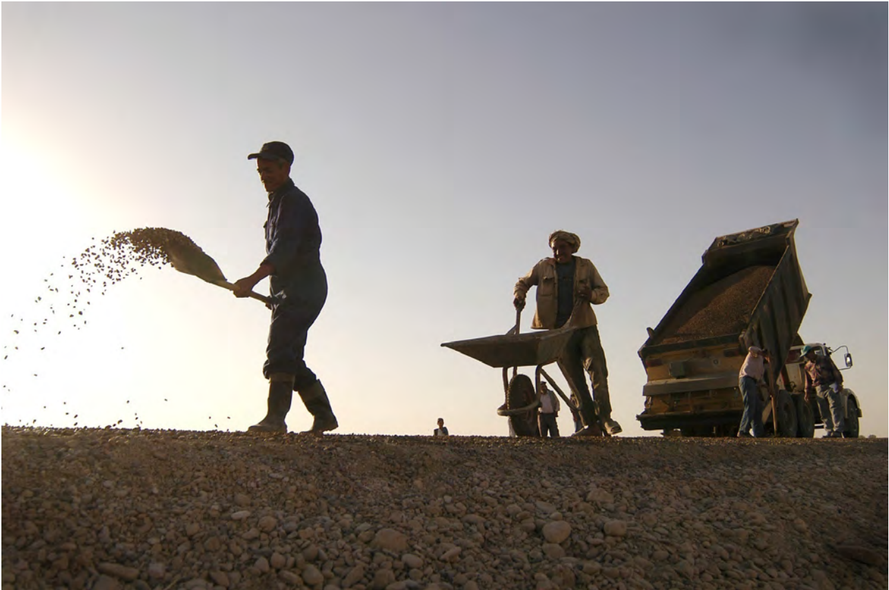
Workers on a road construction site
