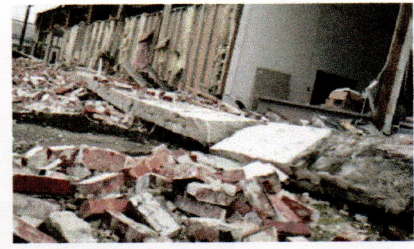
Earthquake damage in Washington in 2001
