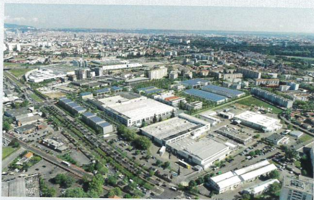
Site Usin Lyon Parilly. © Serl
