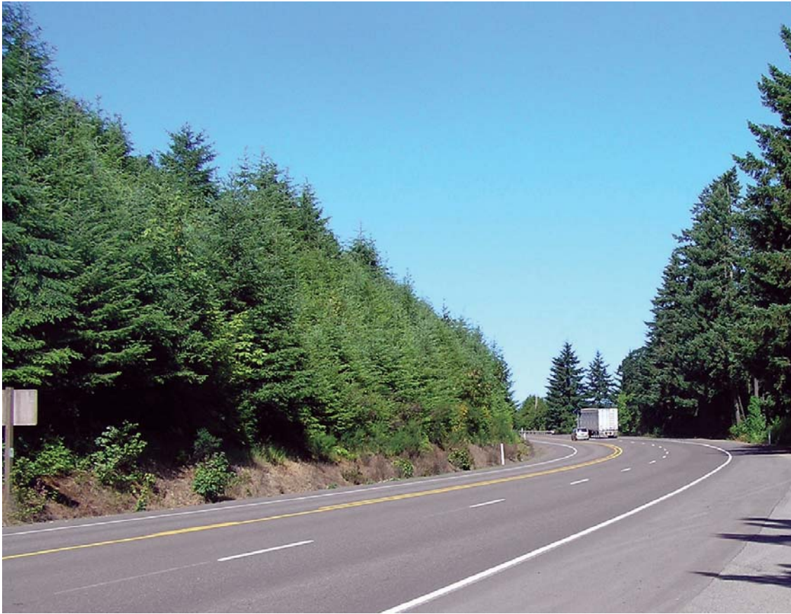
Figure 7-1. Climbing Lane on Two-Lane Rural Arterial
