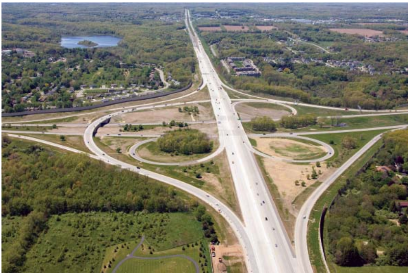
Figure 10-41. Four-Leg Interchange, Cloverleaf with a Semidirect Connection
