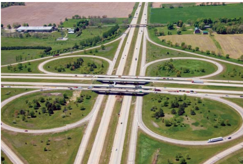
Figure 10-28. Four-Leg Interchange, Cloverleaf with Collector-Distributor Roads
