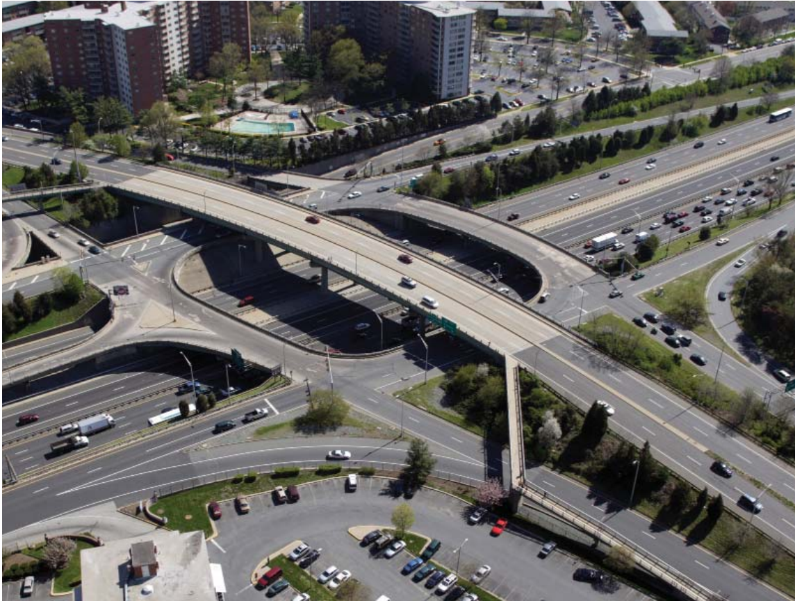
Figure 10-20. Freeway with a Three-Level Diamond Interchange
