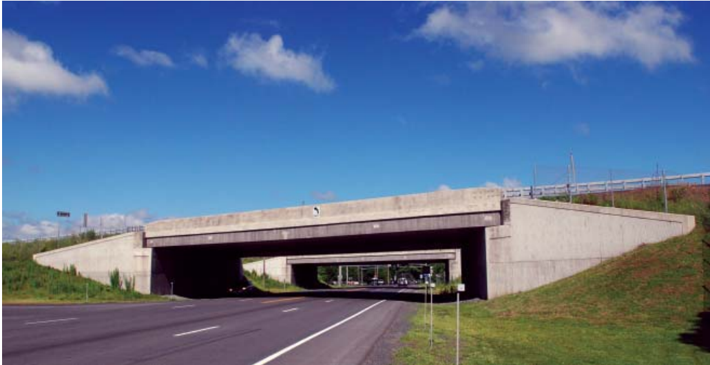
Figure 10-3b. Typical Grade Separation Structures with Closed Abutments
