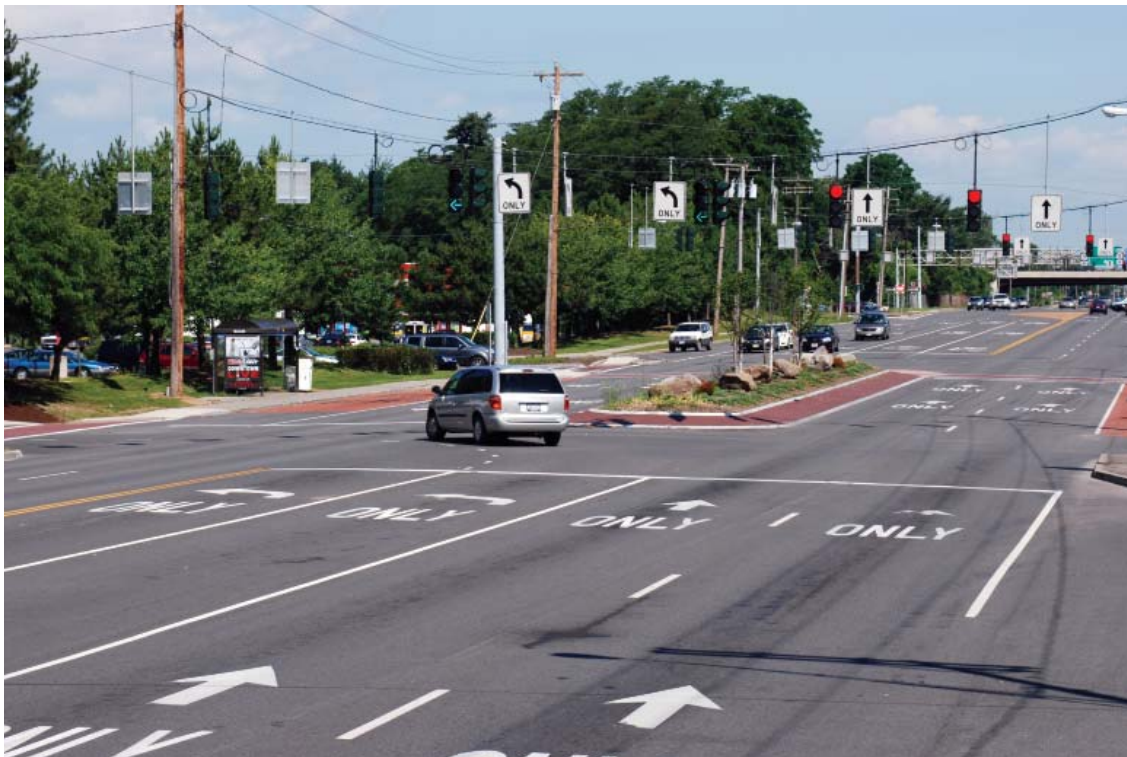
Figure 7-10. Urban Arterial with Dual Left-Turn Lanes
