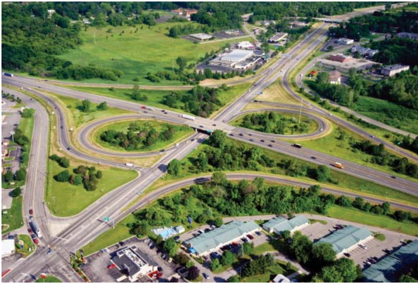
Figure 10-27. Partial Cloverleaf Interchange
