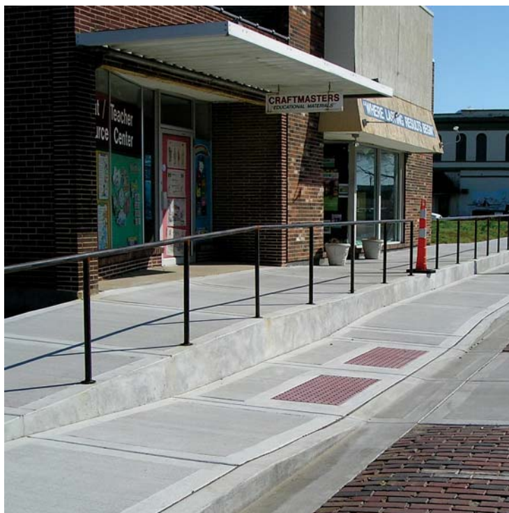
Figure 4-20. Examples of Sidewalk Curb Ramps
