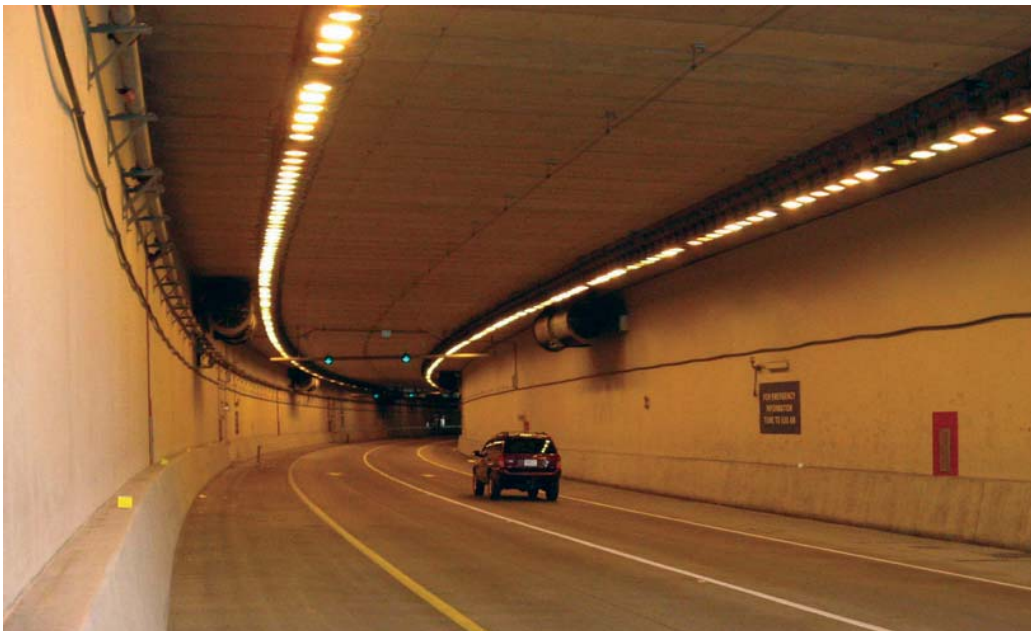
Figure 4-17. Interior of a Two-Lane Directional Tunnel
