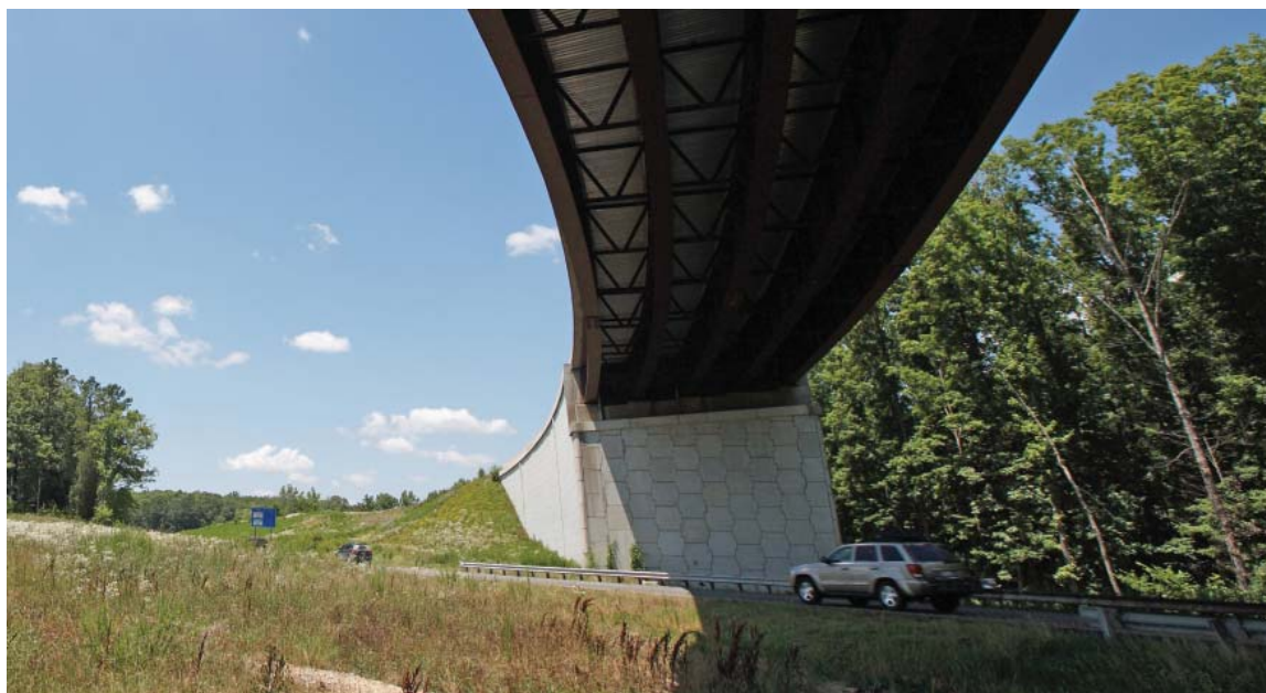
Figure 10-3a. Typical Grade Separation Structures with Closed Abutments
