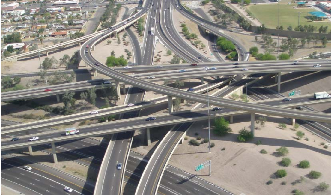
Figure 10-37. Four-Level Directional Interchange
