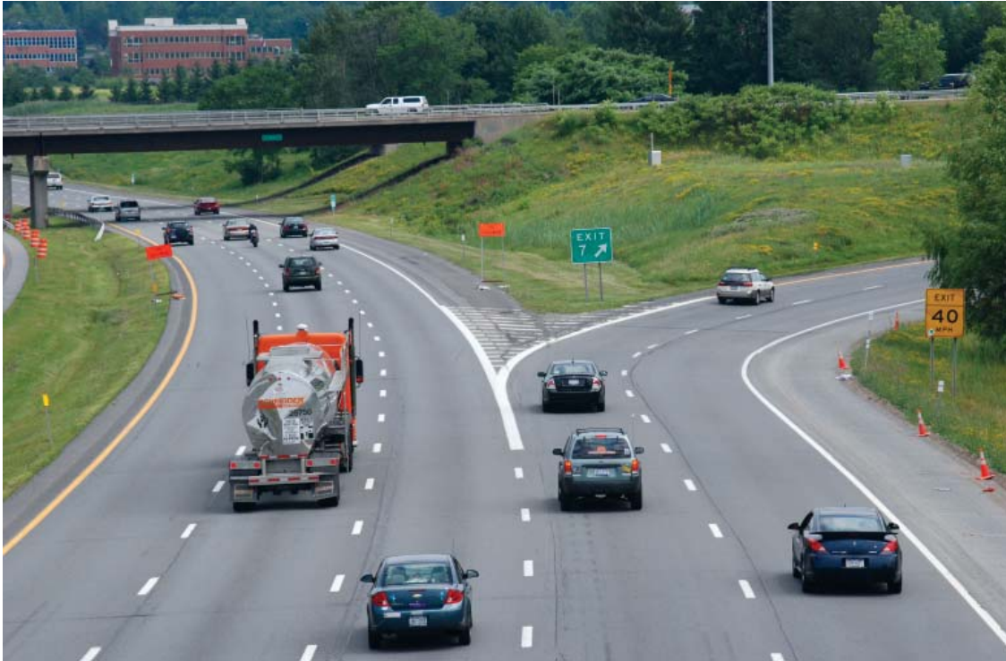
Figure 10-66. Gore Area, Two-Lane Exit
