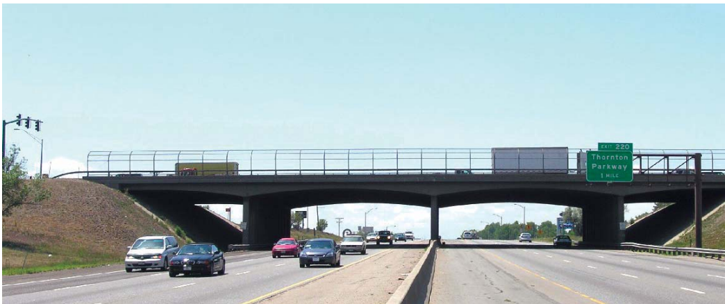
Figure 10-4. Typical Grade Separation Structure with Open-End Span
