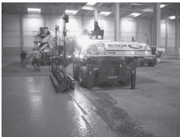
Fig. 50.4 Steel–FRC floor installation. (Supplied by J. Greenhalgh, Bekaert Ltd, UK ( www.bekaert.com )).
