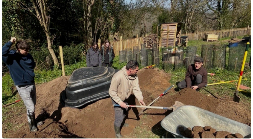
The digging of a hole for the pond. We encountered a large granite boulder that had to be removed.
