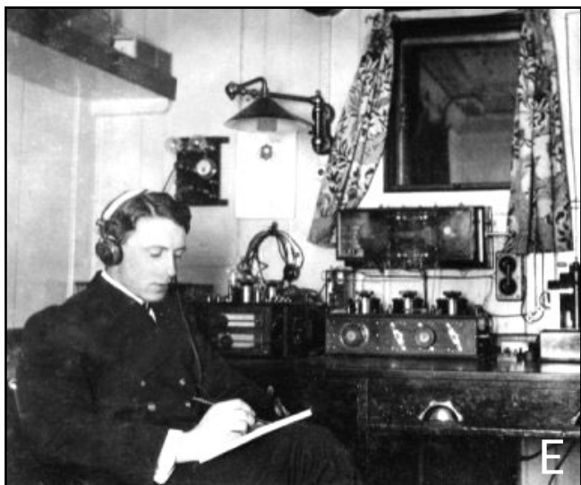
the communication and signal room
