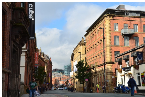
Palazzo warehouses on Princess Street
