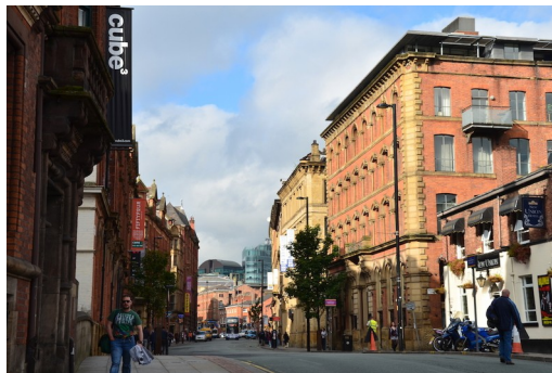
Palazzo warehouses on Princess Street
